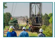
A workover rig arrives on-site. While the rig is on location, the well will be plugged per the plan approved by the COGCC. Cement is pumped into the well to cover and isolate the zones that produce oil and natural gas.
