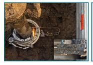
The remaining portion of the well is cut a minimum of seven feet below the surface and an identifying marker is welded to the top of the plugged wellbore.
