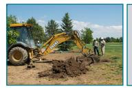
When the plugging operation is complete, the workover rig moves off the location, the well head is removed and the associated flowlines are excavated. Associated surface equipment (tanks, separators, etc.) may also be removed if it is not serving other active wells in the area.
